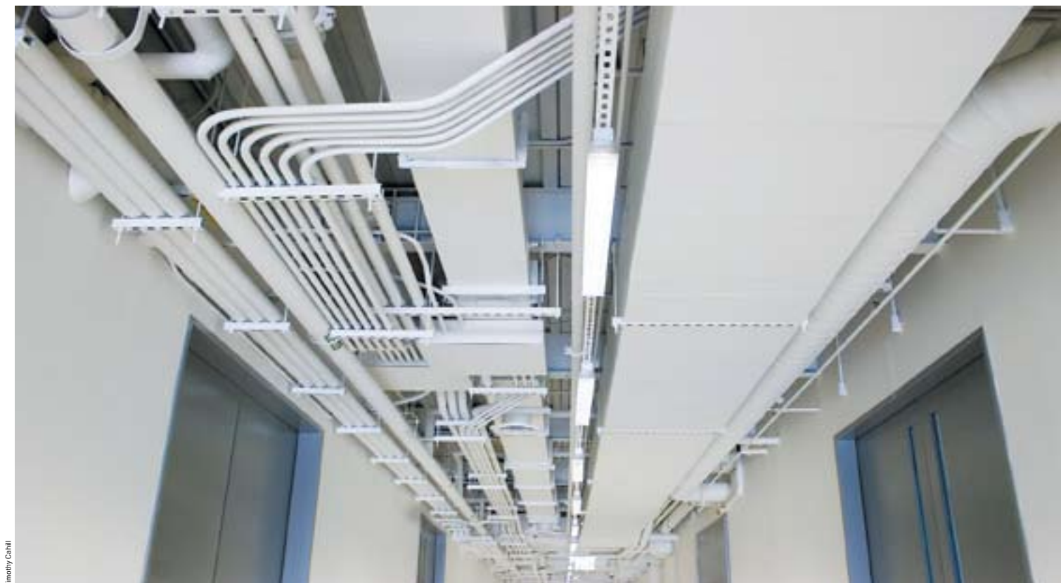
"Our own Louise Nevelson": Exposed pipes, duct work and electrical conduit fitted with precision on the ceiling of WACC's main corridor.
